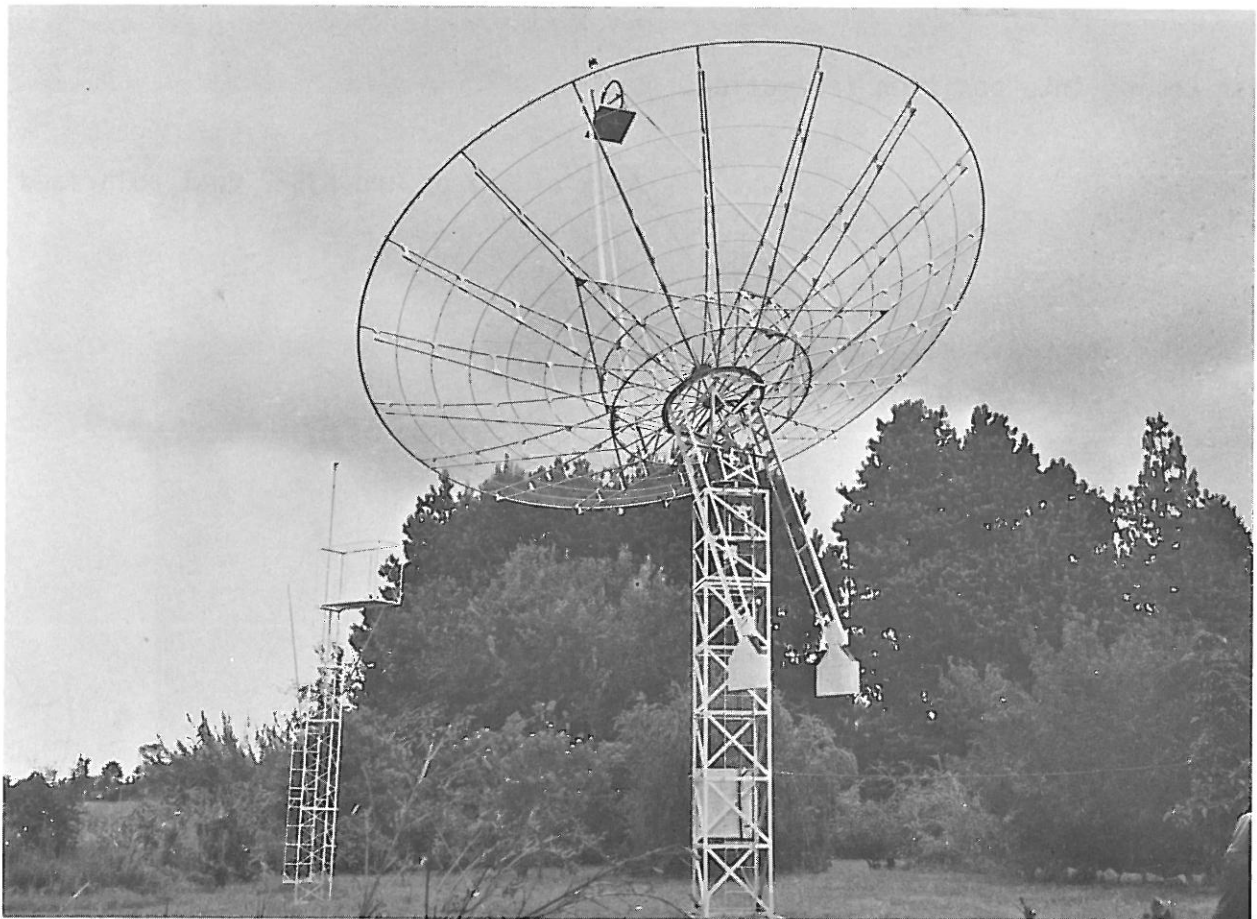
Rear view of complete antenna - note pendulum counter weights.
