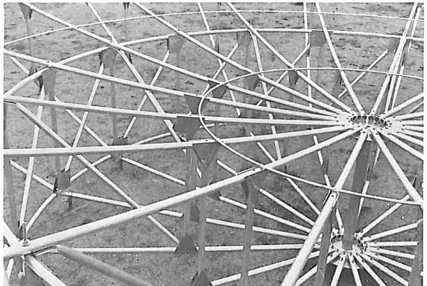
Structure from above showing angular and vertical ties and struts.
