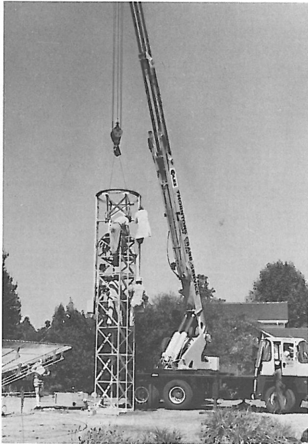
Mating ring assembly integrated with mount.
