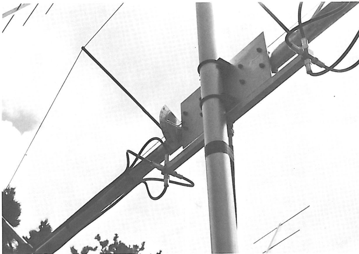
Gusset plate supporting main horizontal boom (25' long). Also shows umbrella support wires (2 planes) to eliminate sag. The 8 port 50 ohm power divider and elevation indicator can also be seen in this view.
