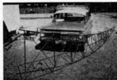
This is one of the more than 20 steel tubing trusses being used in the 50-foot dish at VK3ATN. The 20-foot long trusses weigh 30 pounds each and are within 1/8-inch tolerance of a parabolic curve.
