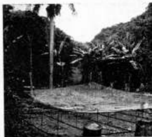
W1FZJ/KP4 is building this 50 foot square "dish" for 432-Mc. e.m.e. tests. The dish will later be expanded to 150 feet for use on 144. A movable feed will be mounted atop a 60-foot tower in the center of the dish.
